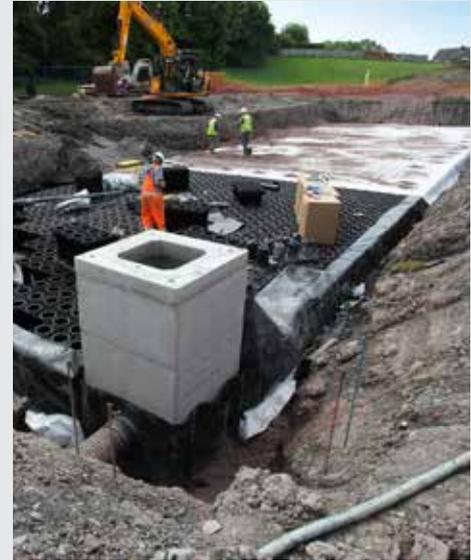
ACO Water Management's ACO StormBrixx system has been utilised as part of an exemplar SuDS design for exceedance. ACO worked closely with the project engineers for Telford Co-Operative Academy, to develop a multi-functional solution able to manage a 1:100 year event plus an uplift of 30% for climate change - equating to around 1000m<sup>3</sup> of surface water.
