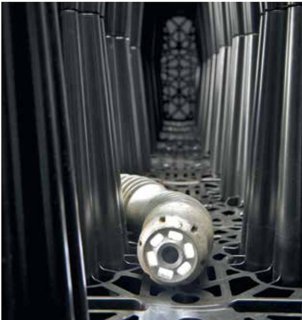
Slide inspection cameras can be easily used in the ACO StormBrixx system.
